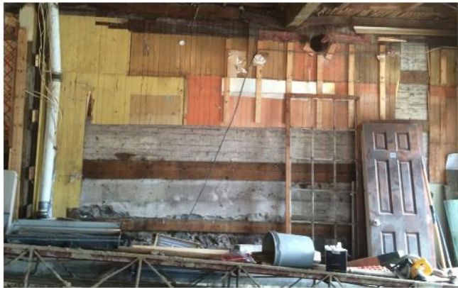
DEMOLITION AT DINING ROOM
